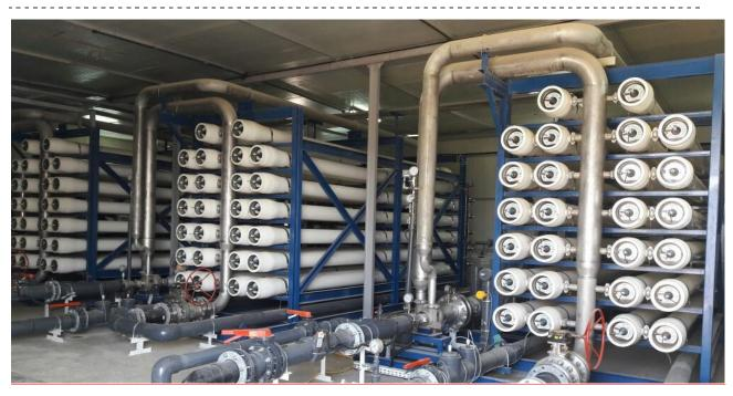
The SWRO series -200 covers applications, industrial application, Potable water; boiler feed water, irrigation and plant process water. For applications with challenging feed water source, combination of multimedia filtration, Ultra filtration can be installed as per the feed water condition.
